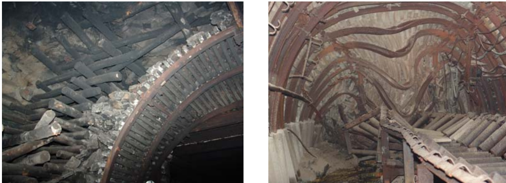
Figure 9: Timbers beyond poling of support Figure 10: Caving in U-24
