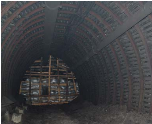
Figure 6: Temporary stopping in U-23
